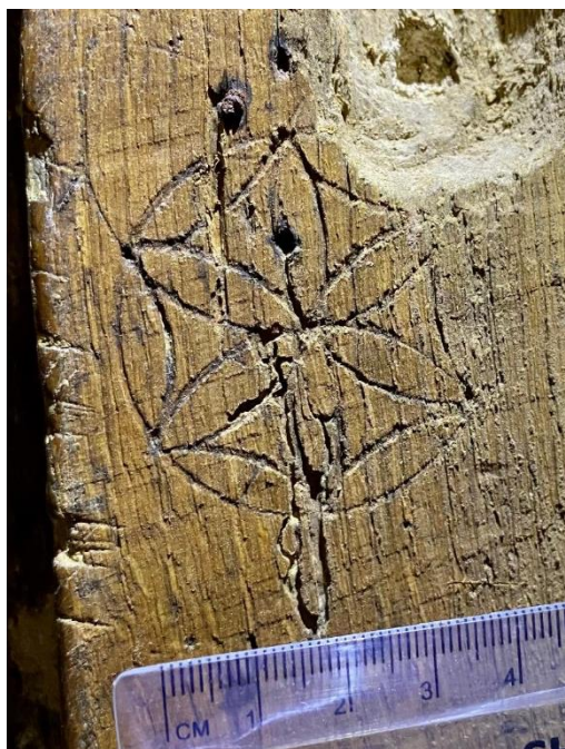
Ground floor parlour, North end
